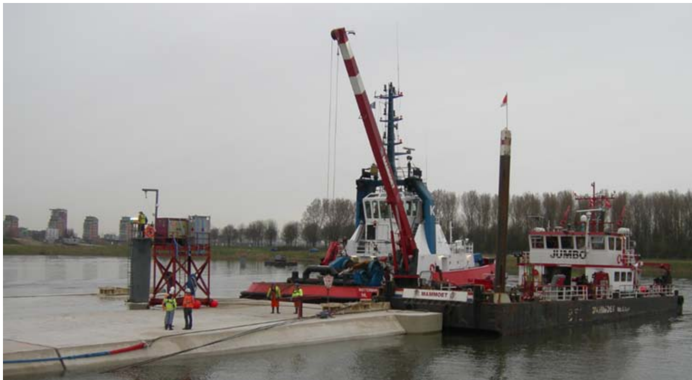
The 3 rd Element (out of series of 4) for the new to built 2 nd Coentunnel was transported from Barendrecht to Amsterdam, above seen Handling the mooring wires before start transport, with assistance of the multipurpose vessel Mammoet JUMBO . The transport was executed by the RT MAGIC as the leading tug, RT CLAIRE stern tug, RT STEPHANY stern tug and pusher tug Mammoet " DIENI ", RT ADRIAAN was connect just before start Nordsea trip Hook of Holland – IJmuiden. Photo : Jos Leentvaar ©
