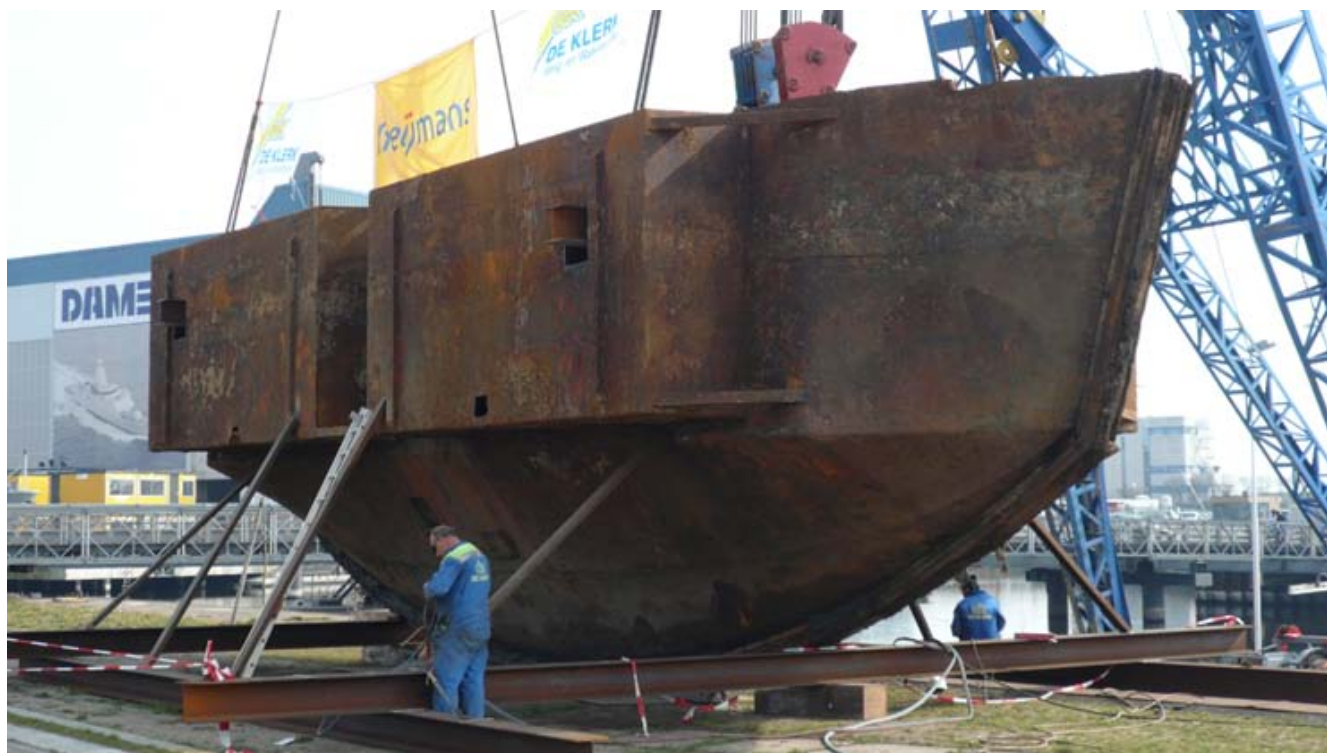
The dock door of the "Dokje van Perry" in Vlissingen was lifted out as seen above - Photo : Huib Lieverse ©
