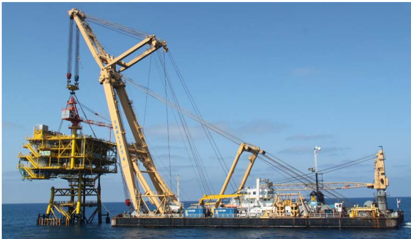
SMIT's shearlegs Taklift 4 installing the 850ton NAQ-PII topside offshore Alexandria, Egypt
