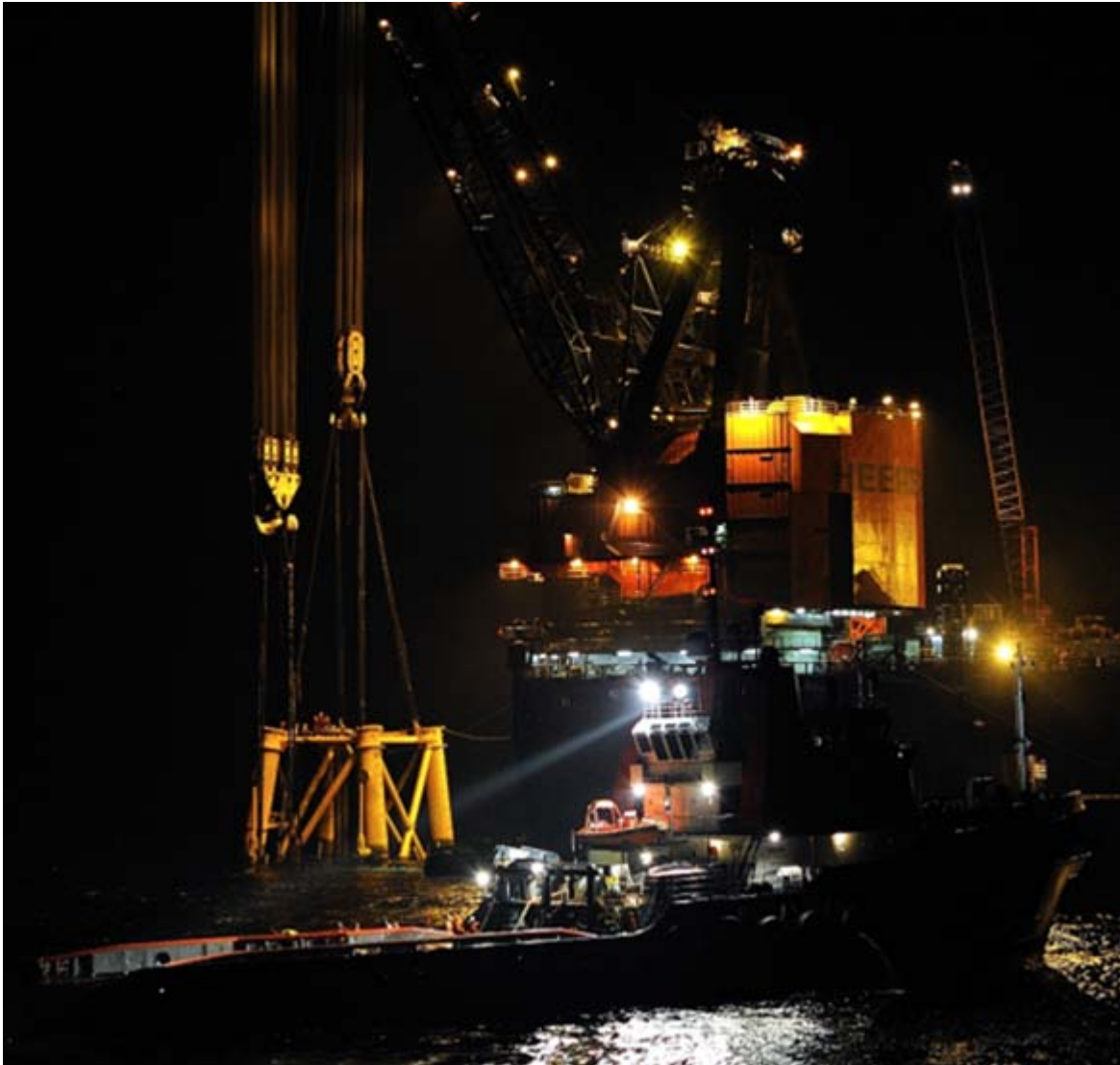
The Hermod seen lowering the Bombay High North N20 jacket to the seafloor. Off course during dark hours. Heerema's tug Retriever standing by in the foreground.
