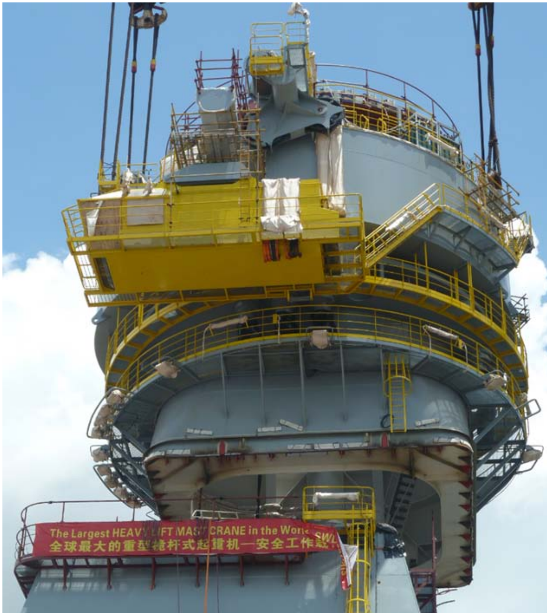
The 1124 tons slewing section for the 5000 ton's HUISMAN crane seen getting installed at the pedestal onboard the BOREALIS in Singapore.
