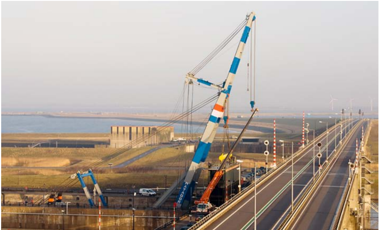
The Bonn & Mees sheerlegs MATADOR seen lifting the 380 tons door of the Krammerlock, to allow the change out of the rollers on the bottom - Photo : Jan Pollemans ©
