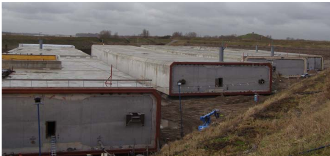
The 4 elements of the new 2nd Coentunnel, last fittings, before filling the building dock at Barendrecht. Transport from Barendrecht to Amsterdam via North Sea, is scheduled in March/April
