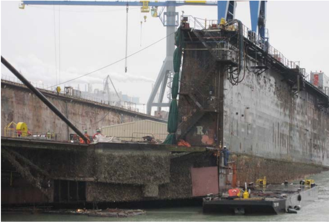
Above seen dock 3 (Panamax) at the Scheldepoort Shipyard in Vlissingen-Oost at present under maintenance away from her original location (quayside E) whilst in the same time the botom is getting prepared before the dock is moved back to her original location - Photo's : F. Bolier ©
