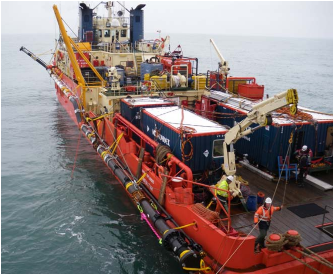
Riser installation at G17 AP from the SEAMAR SPLENDID – Photo : Robin van der Windt ©
