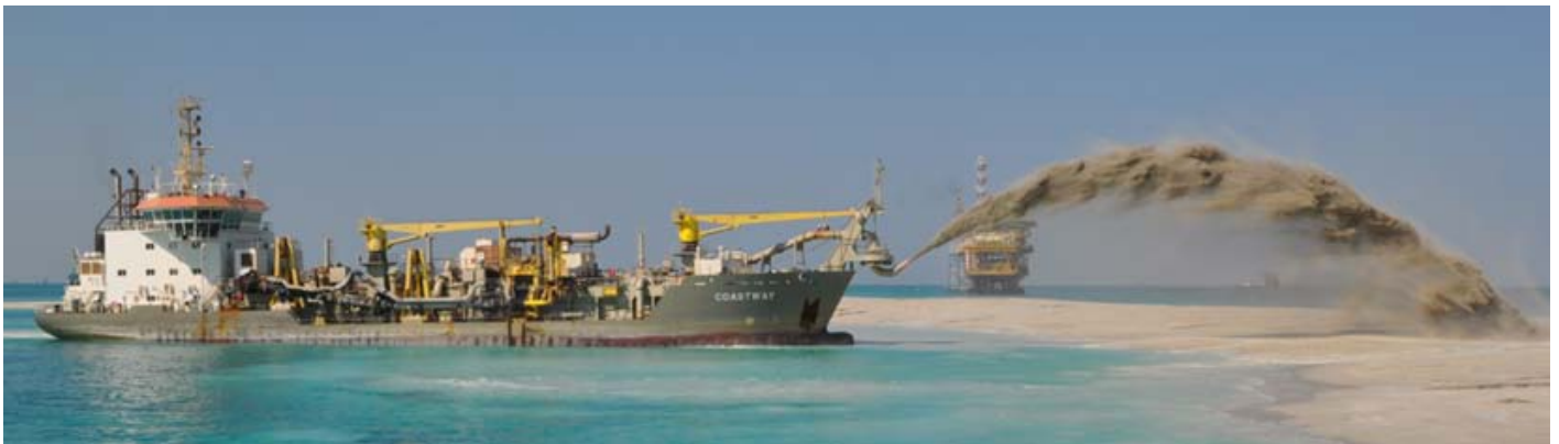
The dredgers HAM 311 and COASTWAY seen during rain bowing at the reclamation of one of the four Upper Zakum Artificial Island 50 miles out of the coast of Abu Dhabi, main contractor of this project is National Marine Dredging Co which receive the contract from Abu Dhabi National Oil Company ( ADNOC ) Photo's : Maarten Mostert
