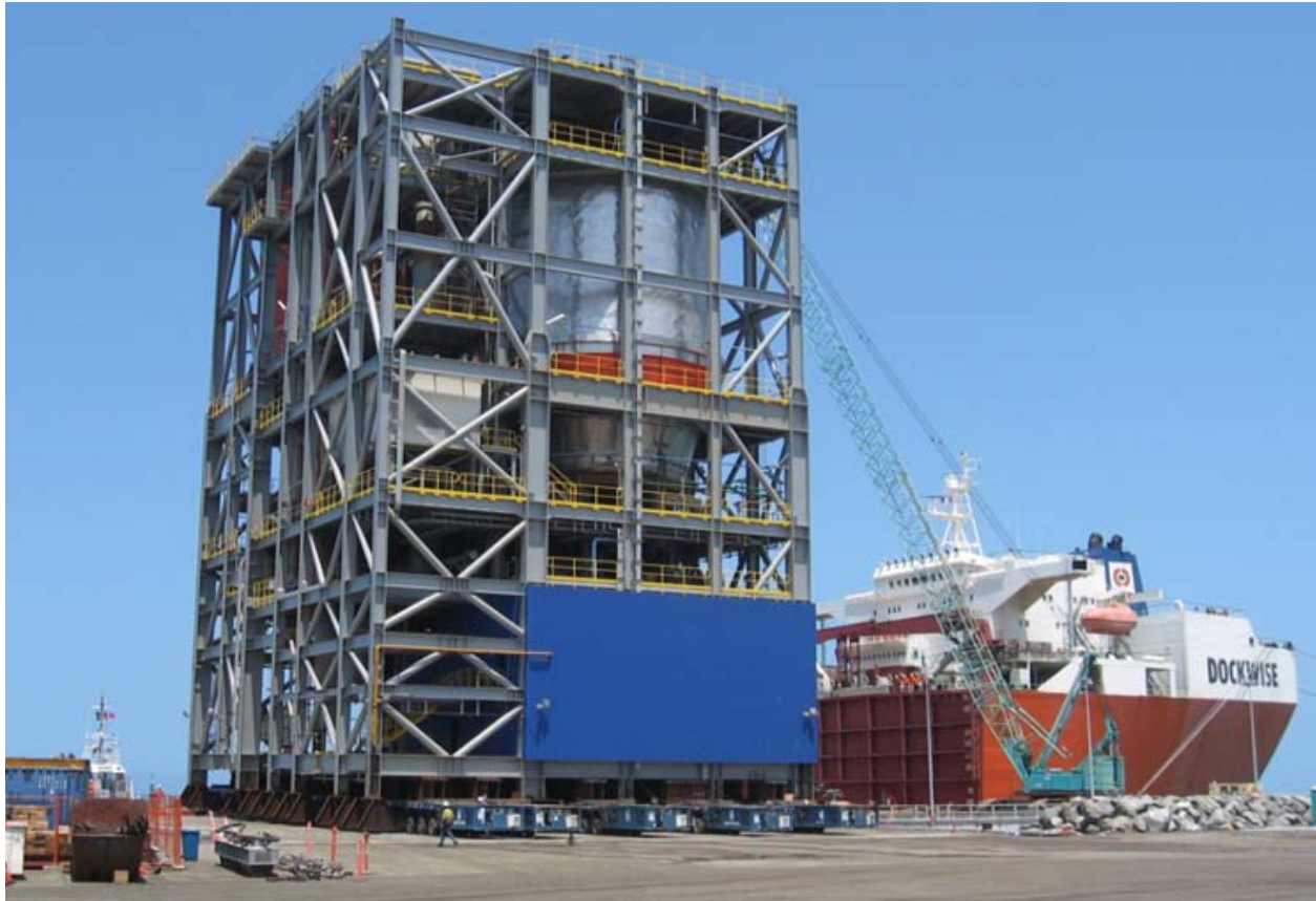
Dockwise Transporter seen off-loading the last of 15 modules. The modules, for a nickel processing plant, were transported in 4 shipments from Qingdao, China, to Vavouto, New Caledonia.
