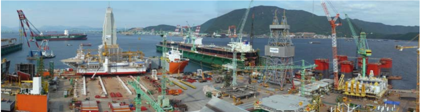
The lower hull and Black Marlin with topside together at Samsung yard. Both are ready for the float over operation.
