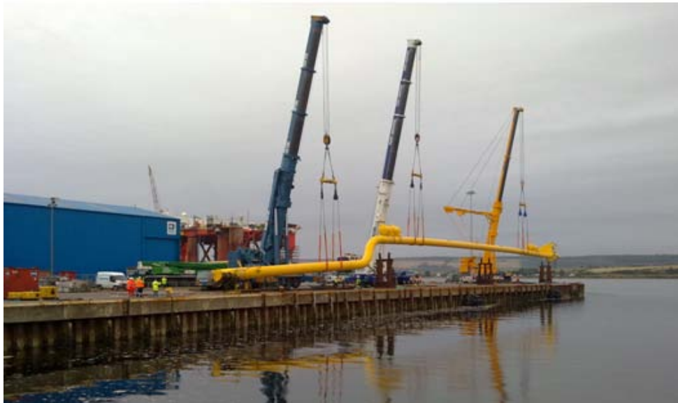
Riser Caisson lifted-in using three cranes.
