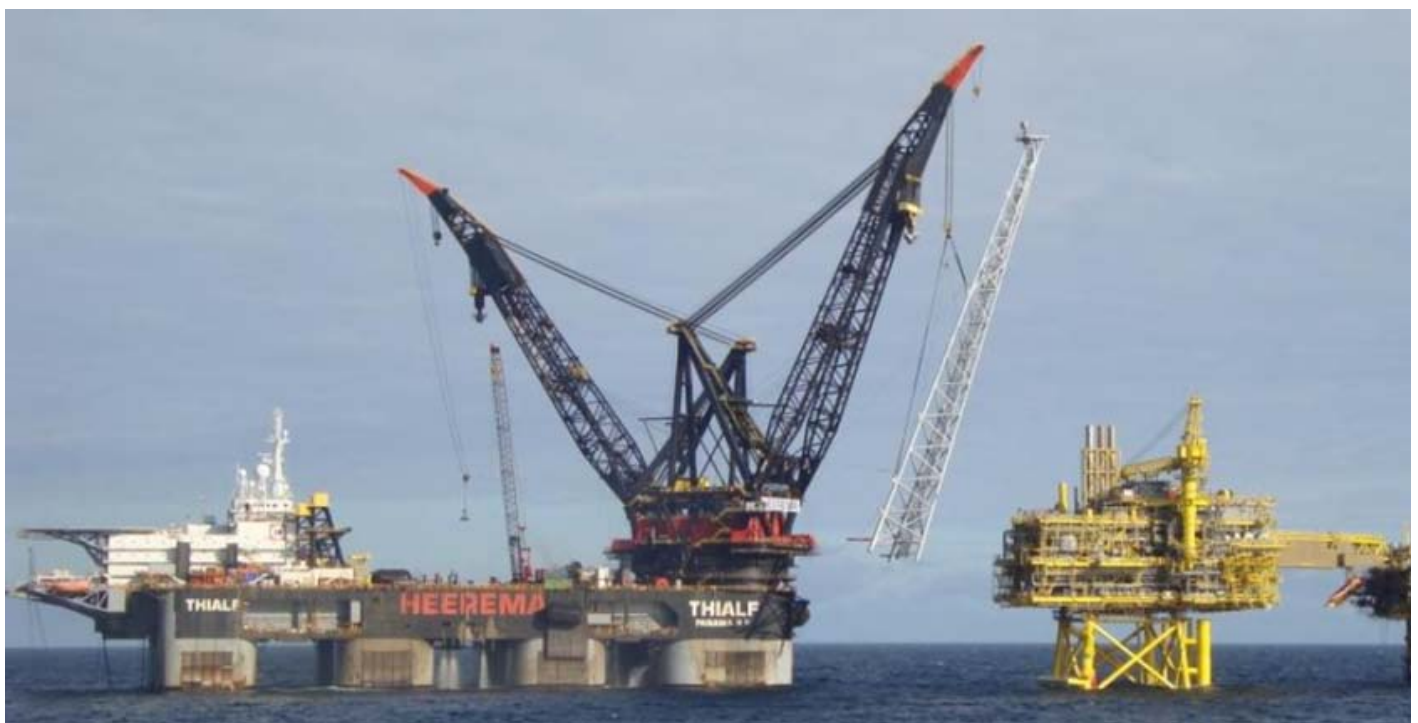
And with the installation of the 110 mtr long flareboom, the Halfdan Bravo - D platform was completed.
