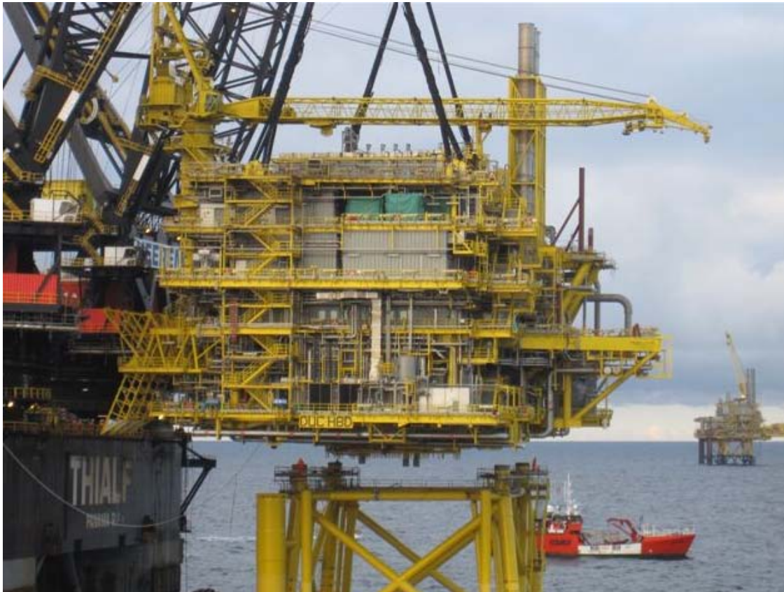
Heerema's THIALF lifted the 9600 ton in weight, HALFDAN D topsite from the FJORD as can be seen above Photo's : crew AHT Taurus (c)
