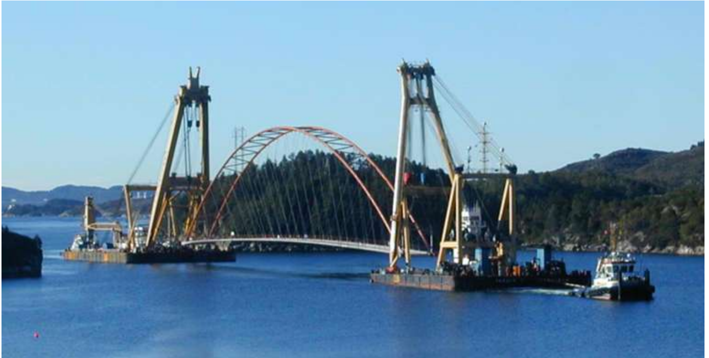
Above seen the installation of the 1862 tons and 220 mtr long Brandangersundet Bridge in Norway near Mongstad bij de shearlegs Taklift 4 and Taklift 7 . Photo : Arie Terpstra (c)
