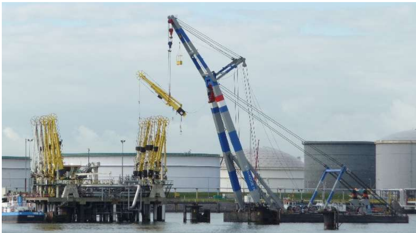
The MATADOR 2 seen last Tuesday installing a new loading/unloading arm at the VOPAK terminal in Rotterdam-Europoort 7 th Petroleum harbour Photo : Jan Oosterboer (c)
