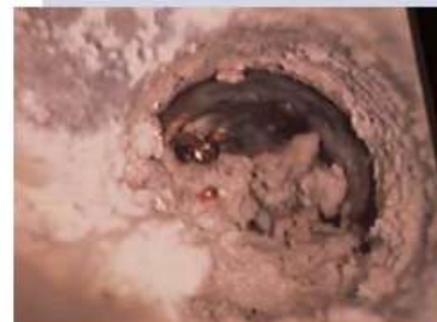
Sediment in the pipe can cause blockage.
