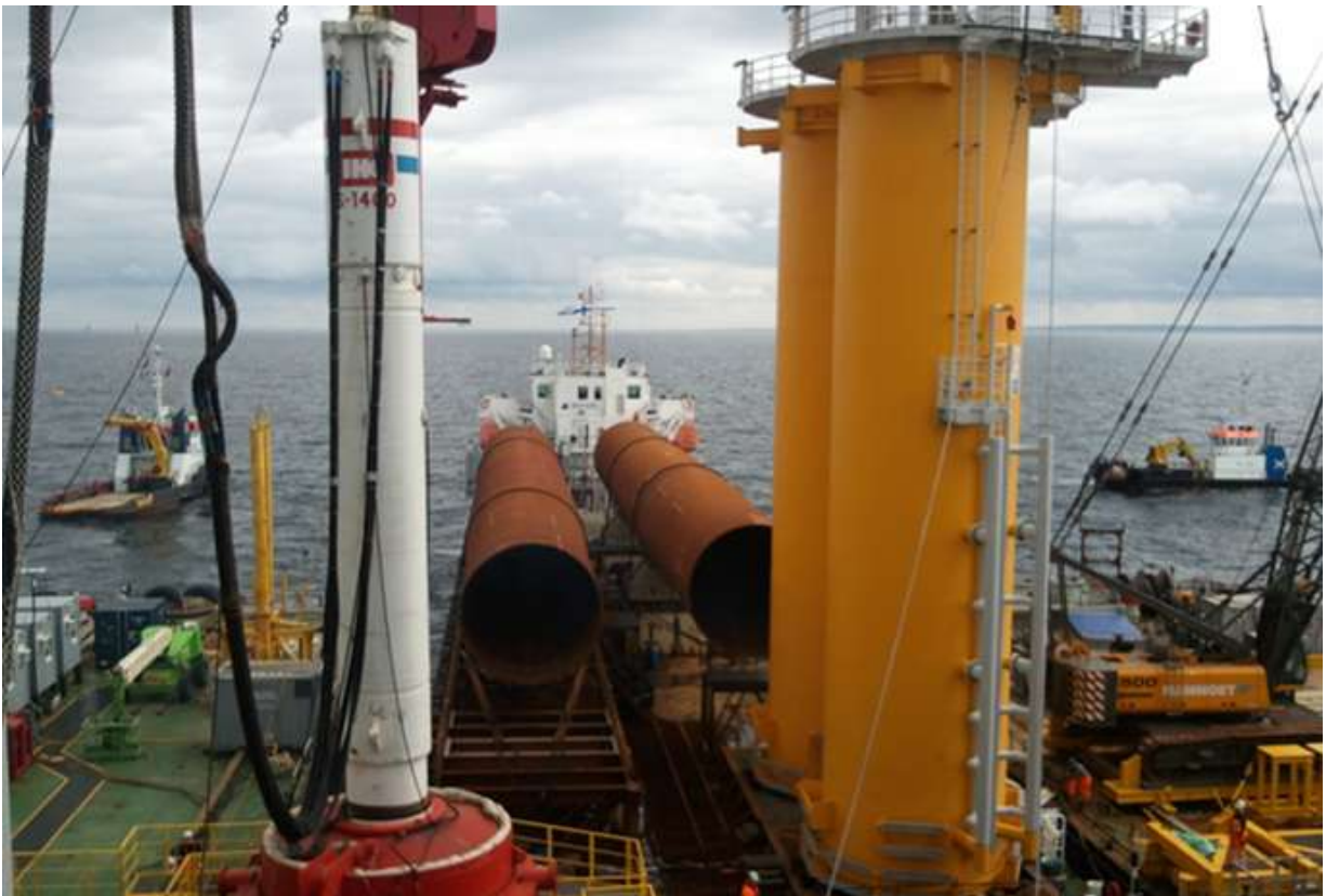
"Dutch Pearl" & "Aileen M" seen guiding "M/V Aura" into the moon bay of "HLV Svanen" delivering mono piles and transition pieces for the construction of the "Sheringham Shoal Offshore Wind Farm"
