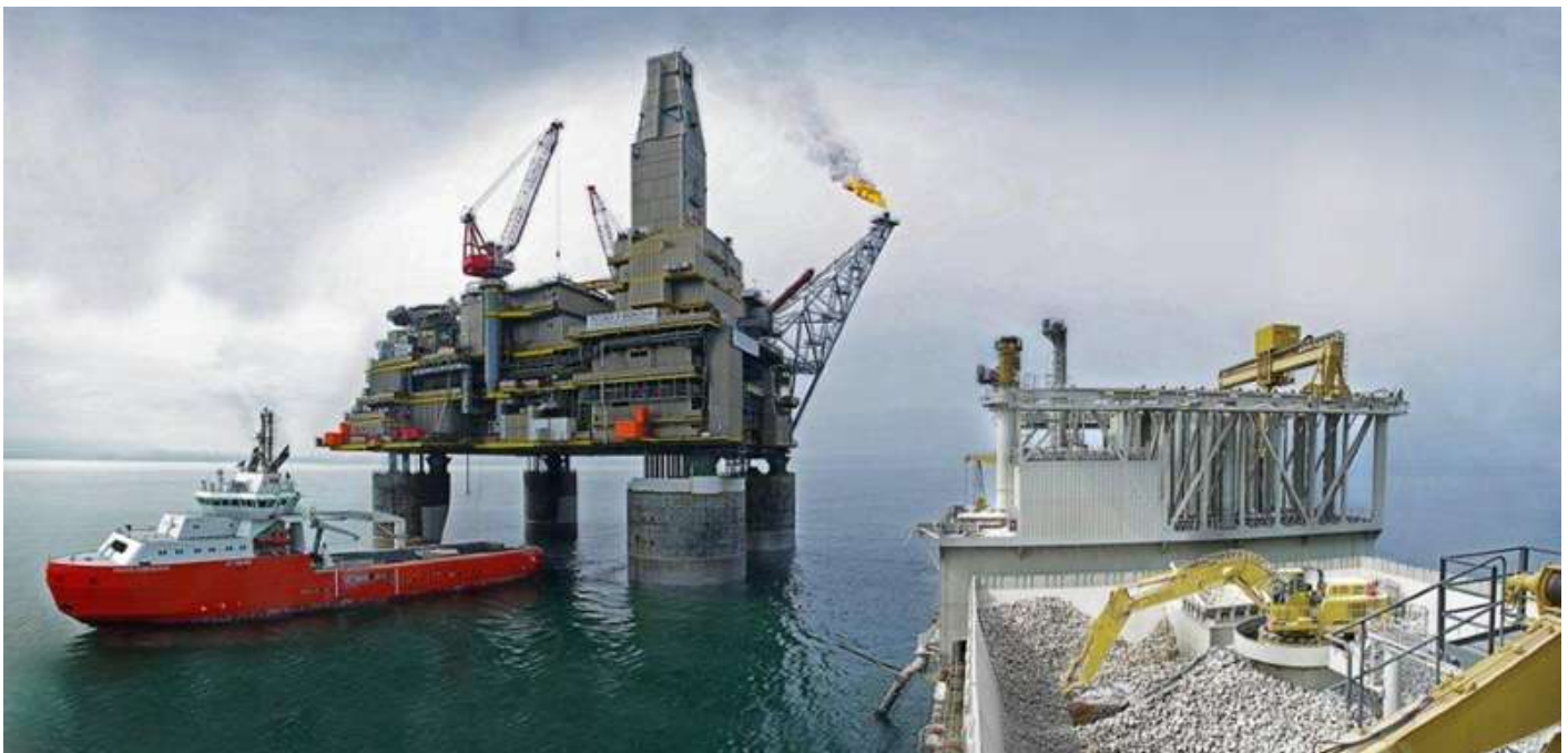
Above and below seen Jan de Nul's SIMON STEVIN operating near the Russian island Sakhalin, the vessel is seen dumping stones / rocks at the foundation of the MOLIPAQ platform and over the pipelines
