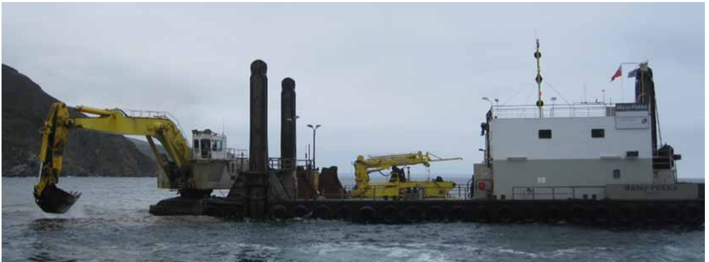
Above seen the Boskalis BHD Manu Pekka , dredging a trench for the Sewage Outfall Project at Polperro, Cornwall Photo : Ferry Hoosemans ©
