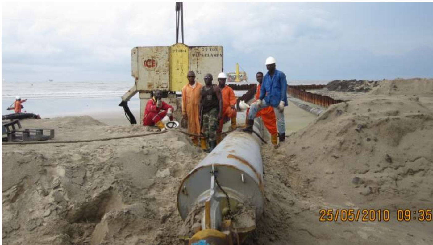
Above seen the final pull of the 24" import line, done by the Van Oord - Boskalis JV , in Escravos, Nigeria. In the background, Clients' (WAV) Lay Barge Jascon-2 can be seen. Photo : Ferry Hoosemans (c)
