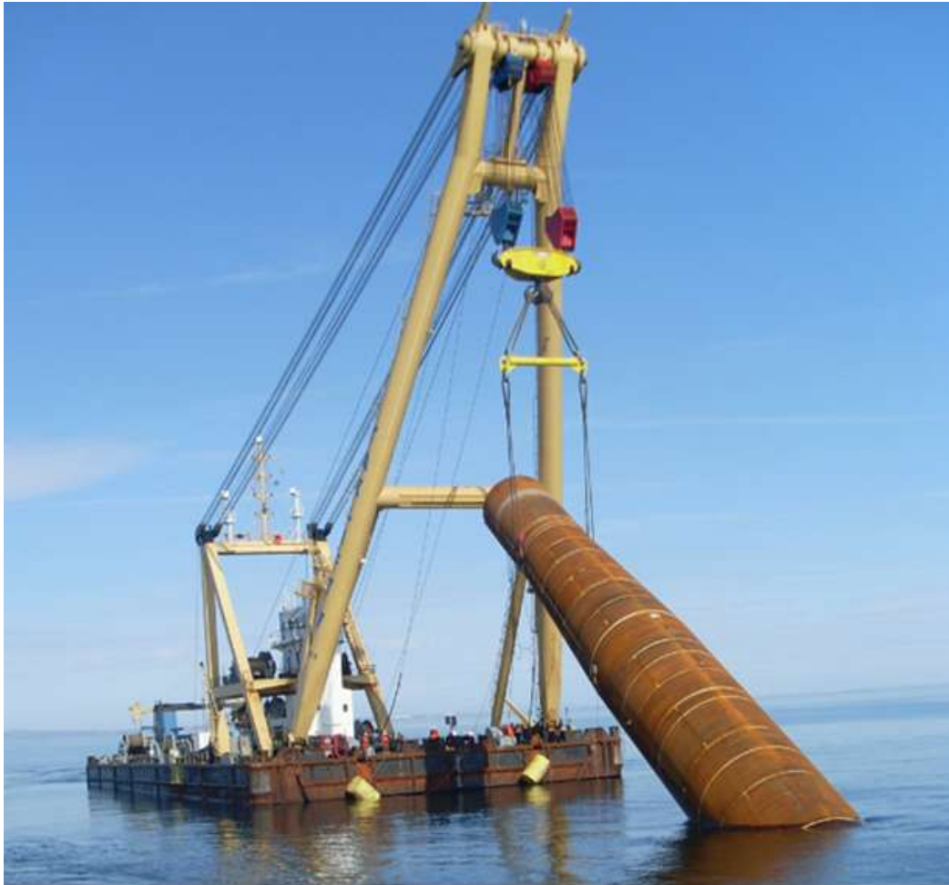
Above seen the TAKLIFT 7 upending 1 of the 51 monopiles off Barrow (United Kingdom)
