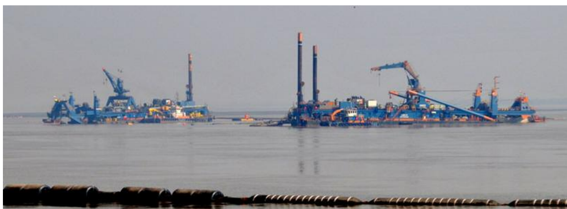
The Van Oord cutterdredgers Castor and Ham 218 seen dredging entrance channel for Essar Plant in Hazira, India .
