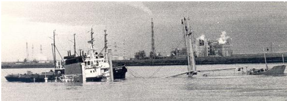
The Wijsmuller tug STENTOR seen by the Marianne Gen , This cargo vessel sank in the River Scheldt, Belgium, in 1973. Ten years later, the wreck was raised by pull barges and sheerlegs
