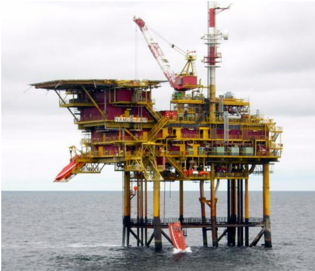
Life boat launch at the L2-FA-1 platform in May 2008. Two of the boat builders are inside the life-boat to test the launch arrangement, the launch was a success!
