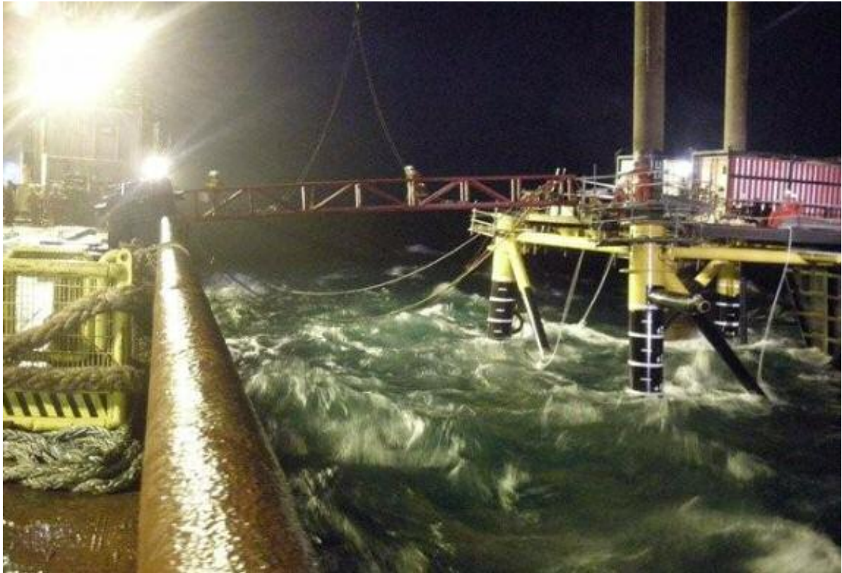
The Stanislav Yudin seen installing West Bukha Jacket in Oman waters .
