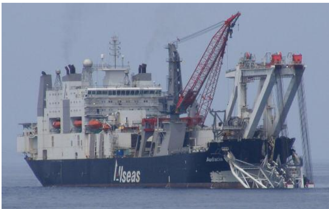
Allseas AUDACIA seen in the pipelaying mode during the Dhirubhai Gas Field development project in India.
