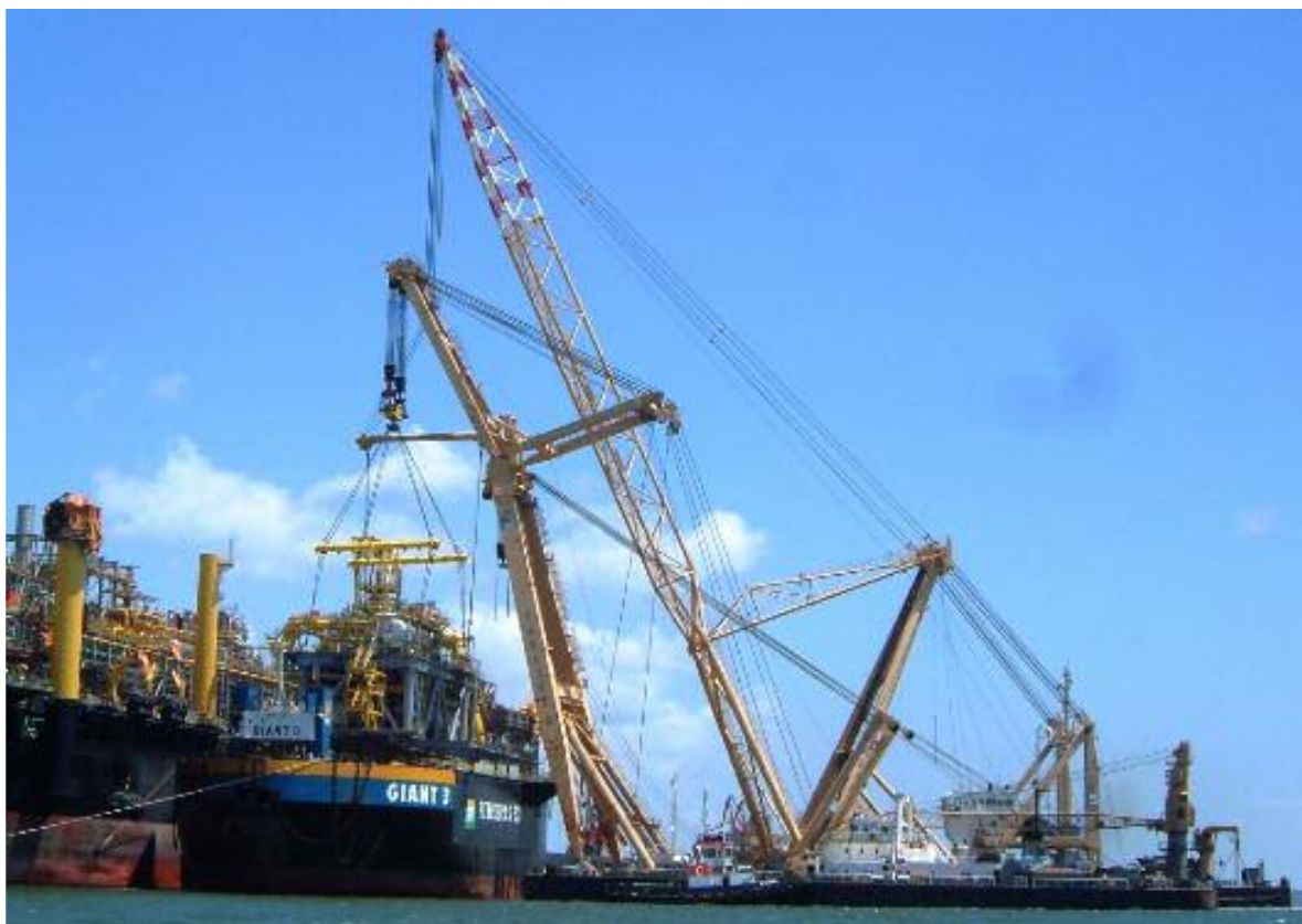
The shearlegs TAKLIFT 4 and TAKLIFT 6 seen lifting the 3 rd module from the Giant 3
