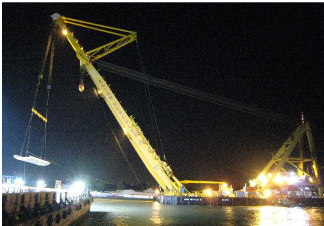
The sheerleg ASIAN HERCULES II seen installing a bridge over the new flood barrier build near Marina Square in Singapore.
