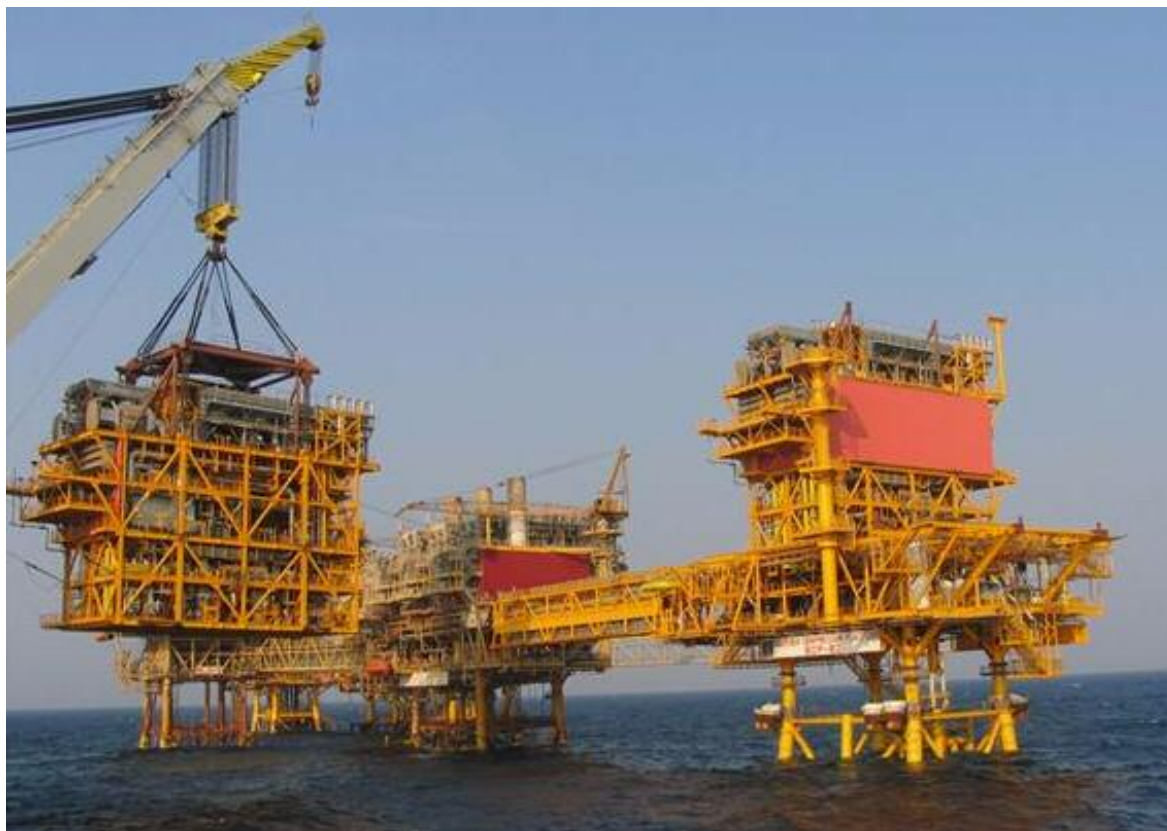
Seaway Heavy Lifting's STANISLAV YUDIN seen lifting one of the two 1800 Tons compressor modules Booster Platform for ONGC India
