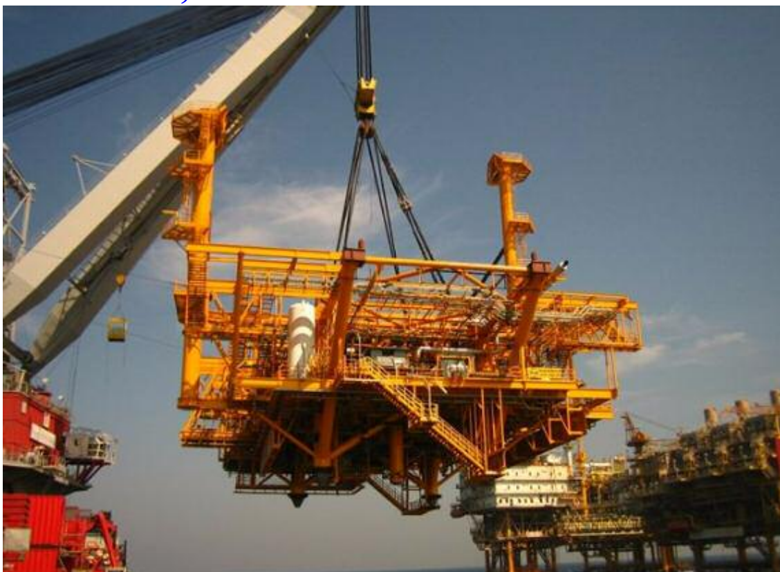
The 2200 ton Celler deck for the Booster Platform (offshore Mumbai) seen lifted in position by the STANISLAV YUDIN
