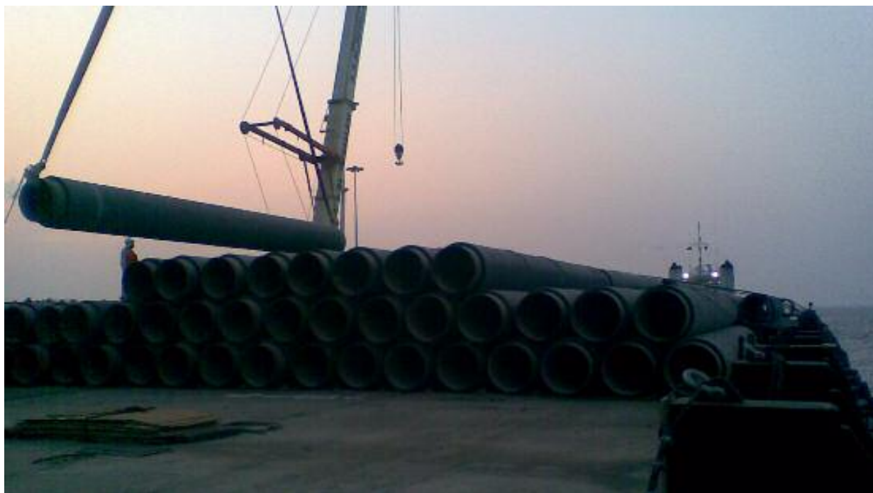
The Barge GT0283 during pipe-loading, Al Khafji Project, Saudi Arabia, transport by CPC Singapore Photo : Udo Borger - Consolidated Pipe Carriers Pte Ltd ©
