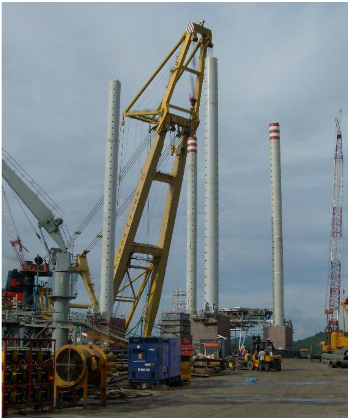
The sheerlegs ASIAN HERCULES seen installing the last leg at the newbuilding Platform JB 109 in Batam (Indonesia)
