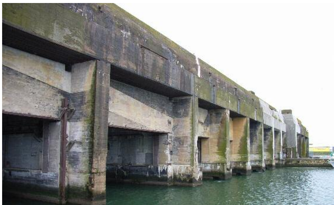
In La Rochelle a Submarine pen can be found as seen above, A submarine pen is a strong enclosure to protect naval submarines from air attack.
