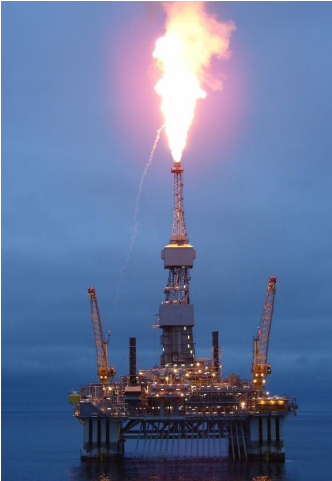
The Flare of the NJORD-A was lighted for the first time using a flare which was shoot through the gas cloud.
