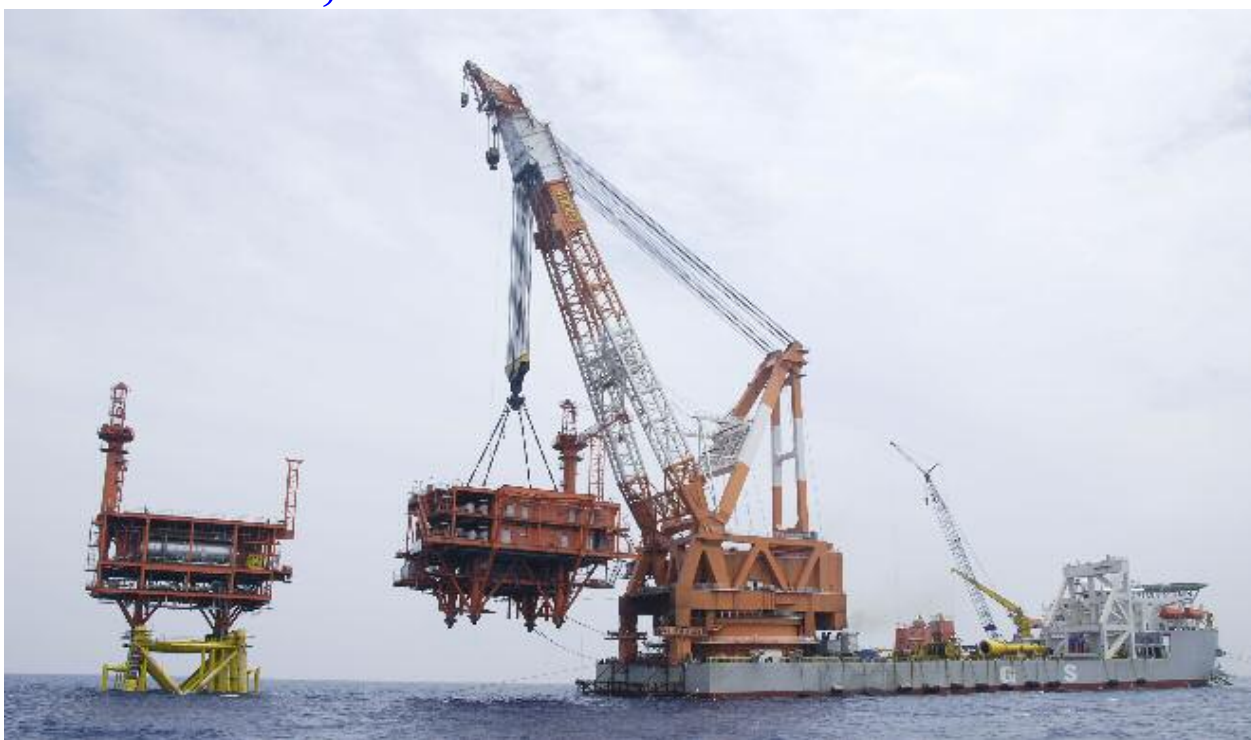
The first two big lifts of the HTL4000 seen above, the first lift was 1680 tons and the second one was 2330 tons. Photo : Li Chang ©
