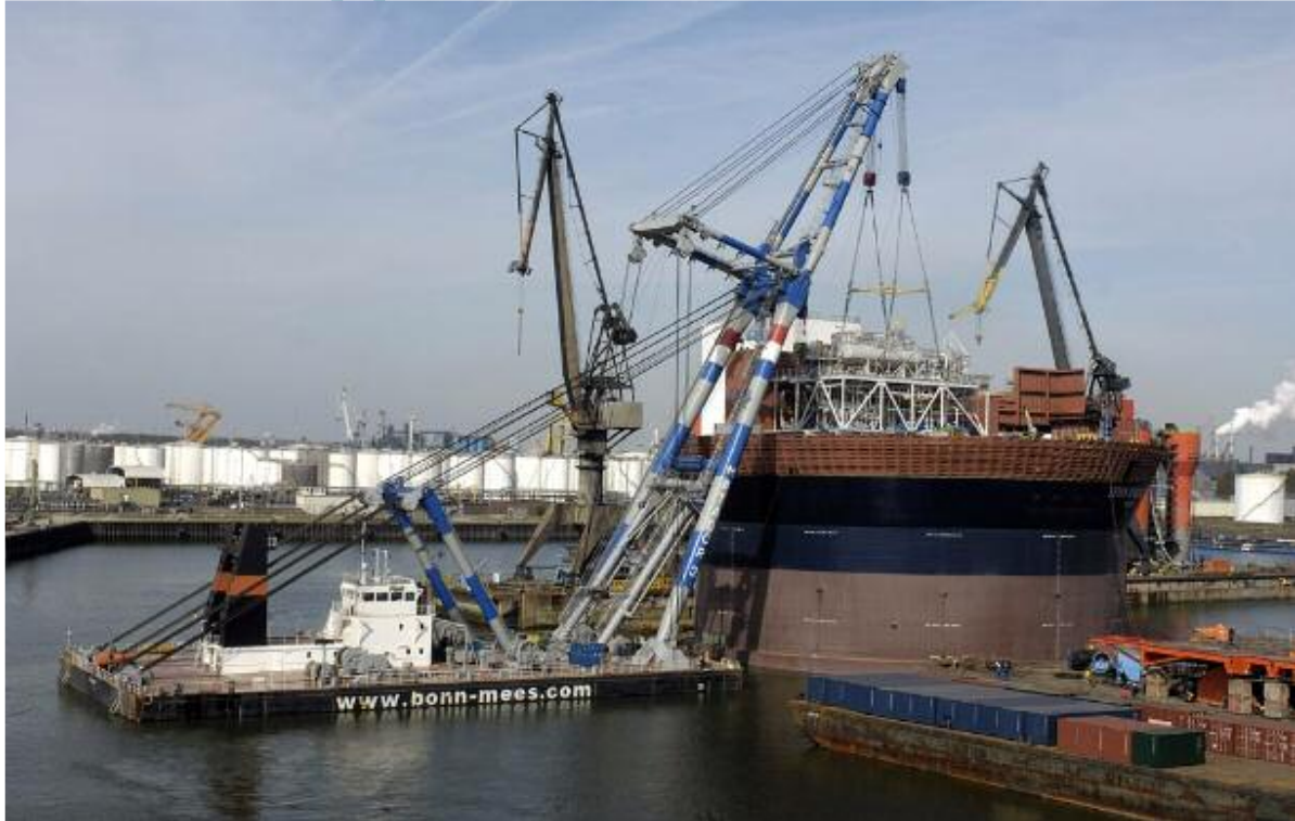
Bonn & Mees Sheerlegs Matador 3 installed the first module on the top of the FPSO Sevan Hummingbird at Keppel-Verolme Yard in the Botlek, Rotterdam. The weight of the module was around 350 tonnes.
