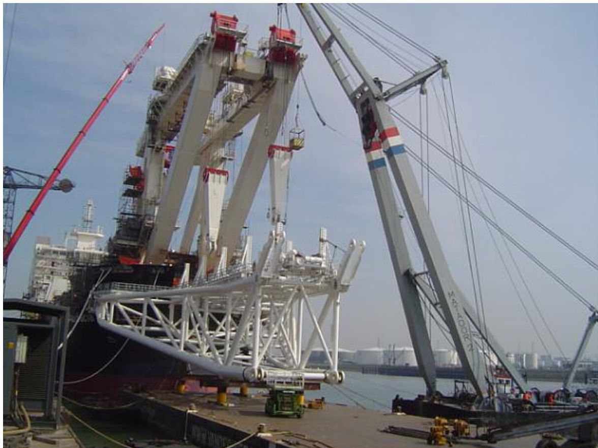
Installation of the new stinger at the AUDACIA at Keppel-Verolme by the sheerlegs MATADOR 2 Photo : Kok Muijsson ©
