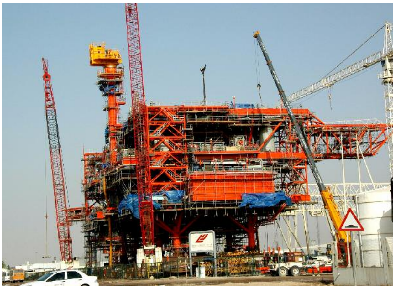
Large top-site section under construction at Lamprell Energy in Jebel Ali
