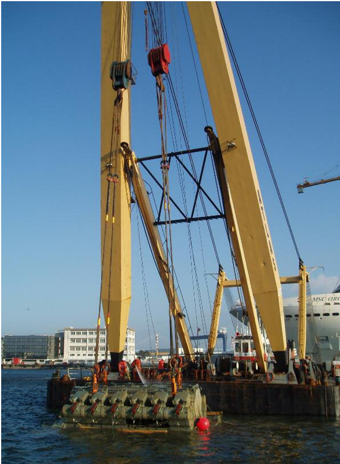
GPS Marine Services BV of Sliedrecht salvaged a lost ships engine at port of Saint Nazaire. The engine was lost during heavy lift operations of m/v Lilleborg in December 2006. The engine was successfully recovered by the sheerleg GPS Atlas .
