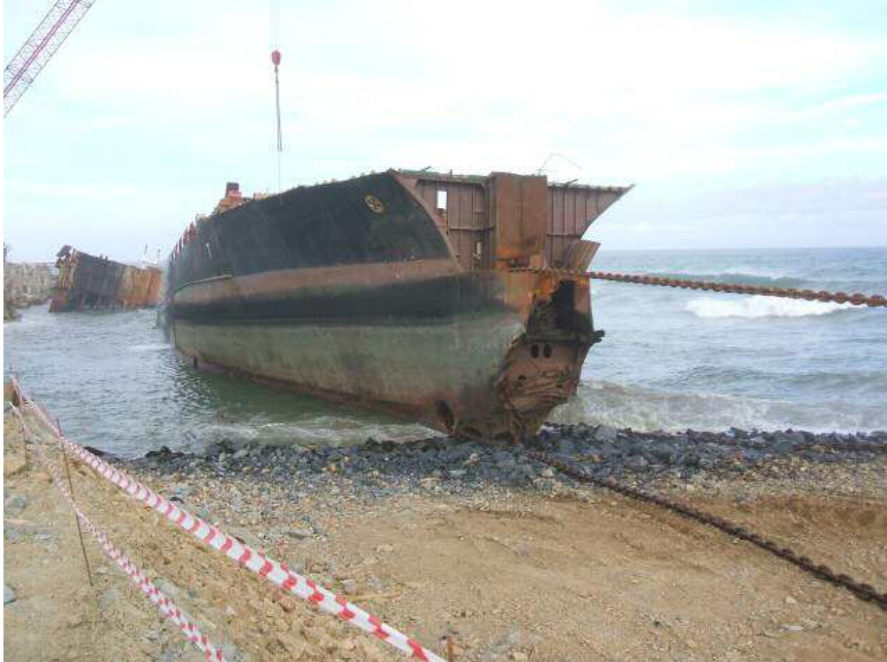
Chain pullers seen pulling the bow section ashore of the SAFMARINE AGULHAS in East London. Photo : via MAMMOET Salvage
