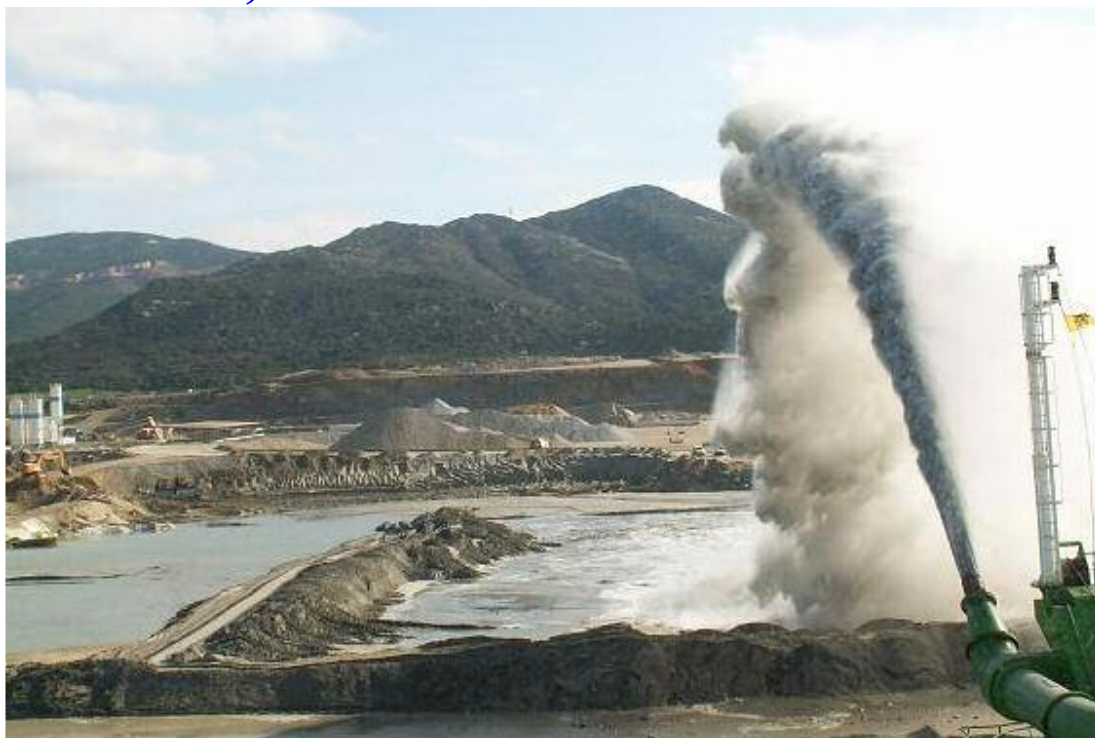
The UILENSPIEGEL seen rain bowing during works in Tanger (Morocco)
