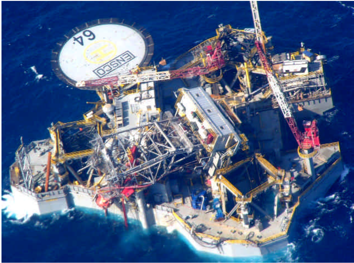
The jack-up rig ENSCO 64 in the Gulf of Mexico after the hurricane IVAN had passed
