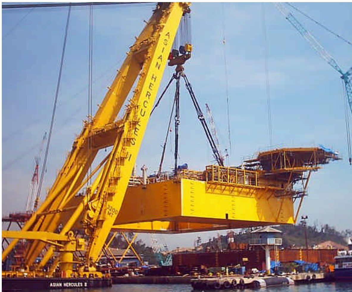
Top : The sheerlegs ASIAN HERCULES II seen here recent carrying out an operation for Nippon Steel Batam. The project was for Bass Gas. The lift in the picture is a 2700t Deck. The deck was lifted off and to be integrated to the Base Structure. During this operation a 1600mt jacket was also lifted and up-ended by the AH II utilizing the Fly Jib and Main frame. The Jacket was subsequently integrated to the Deck and Base Structure. The Asian Hercules II we will be returning for the last phase. Photo : via Eric Ang – Asian Lift ©
