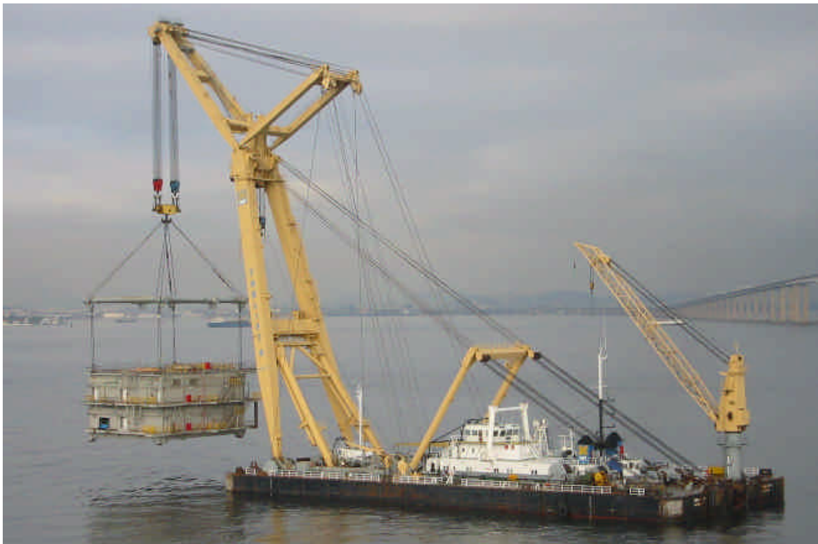
The sheerlegs TAKLIFT 4 lifting a module in Rio de Janeiro – photo : Albert Snoei ©
