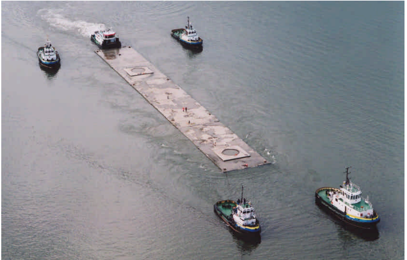
Saturday morning early the 2 nd Element for the new to build Dordtsche Kil tunnel was transported from the building dock in Barendrecht to the construction site – photo : HSL Drechtsesteden ©
