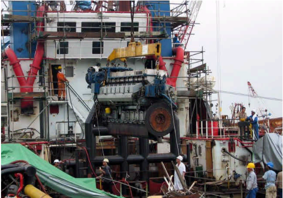
Top : Lifting out one of the main engines
