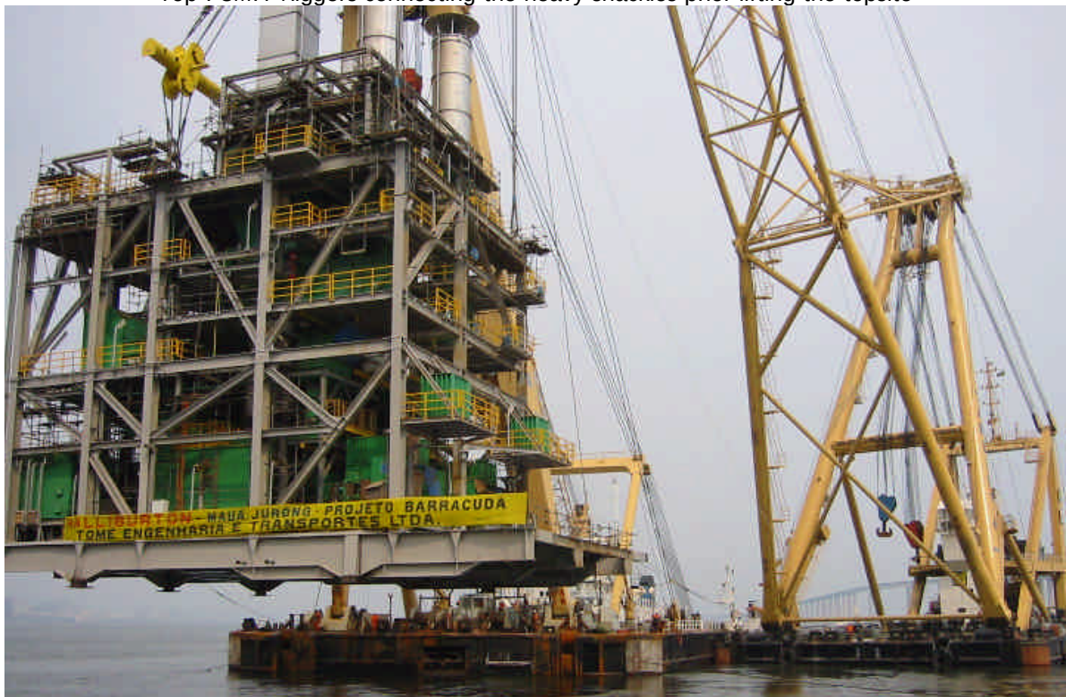
The topsite lifted by the shearlegs TAKLIFT 4 and TAKLIFT 6 Photo's : Albert Snoei ©
