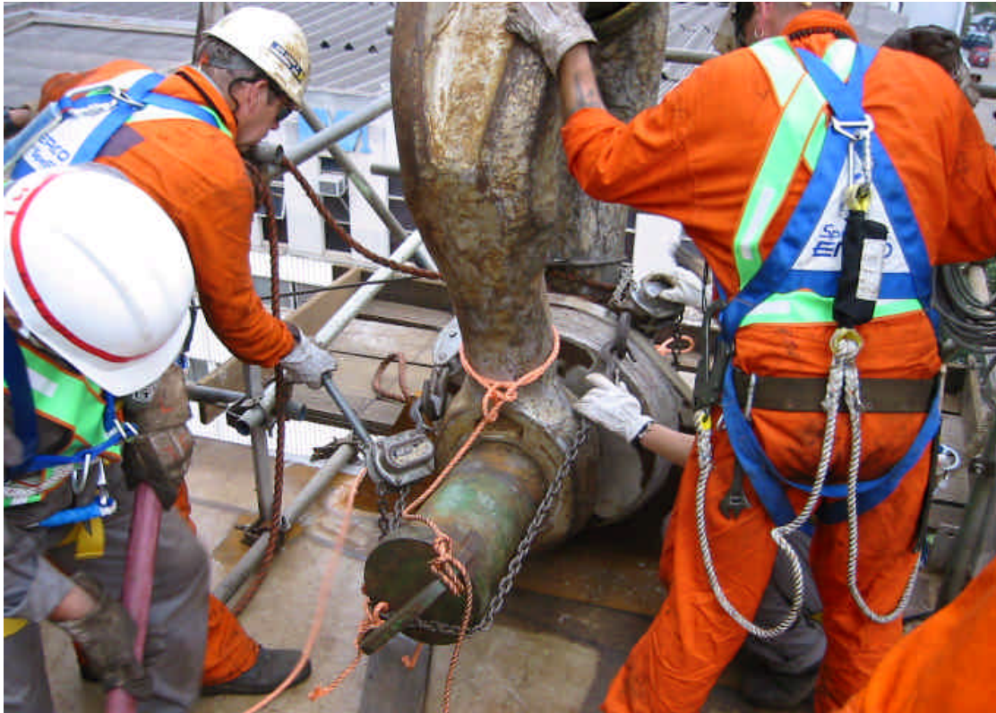
Top : SMIT Riggers connecting the heavy shackles prior lifting the topsite
