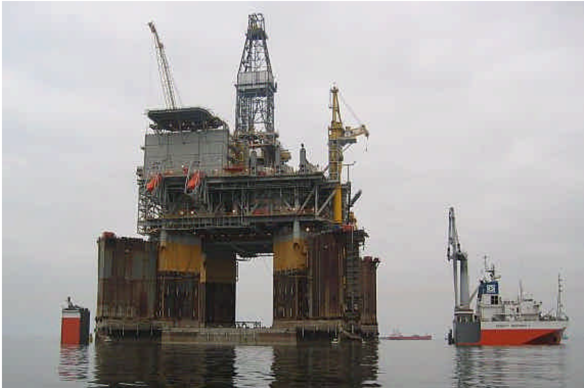
The KIZOMBA-A platform was floated-off the Mighty Servant 1 offshore Luanda
