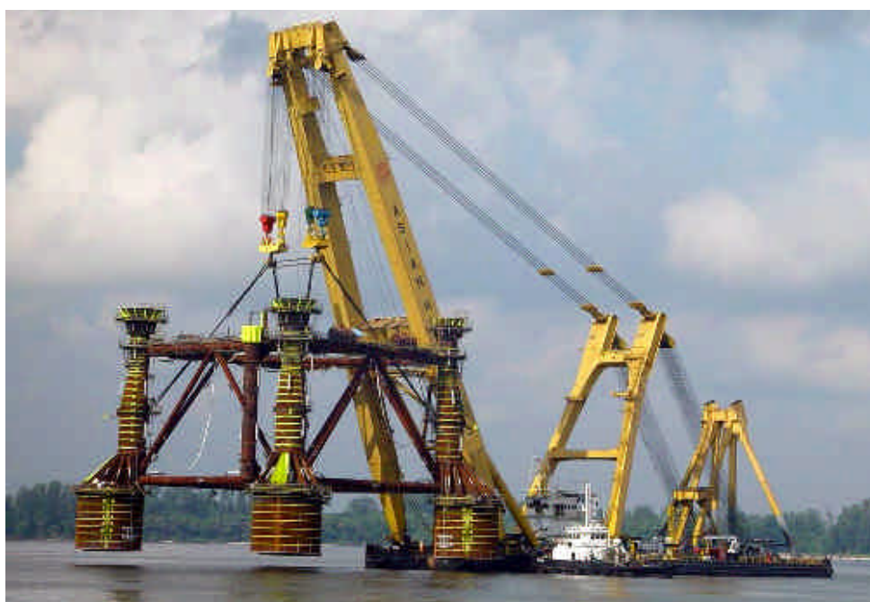
The ASIAN HERCULES ( 1600 tons capacity ) lifted the 1400 tons Talisman substructure into the water at Johore, Malaysia Shipyard and Engineering. – photo Jaap van Heeren ©
